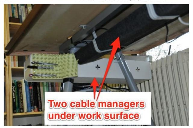
The second cable management system is perpendicular to the white box, and consists of the dark felt trays with the light brackets holding them to the underside of the work surface. IKEA has apparently killed both these cable management systems, but fortunately, they have introduced new systems as well. So, for \$40 you can have all the under-work surface cable management you need.
